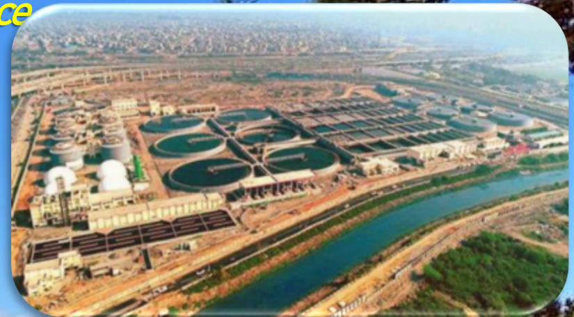
Wastewater Treatment Plant at the Coronation Pillar site in north Delhi
